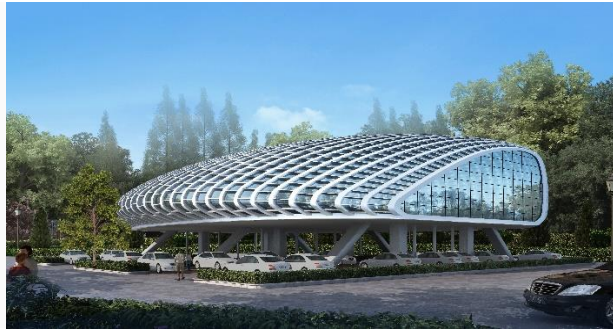
New Tellus DC Supercharging Stations, Beijing
