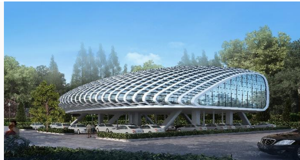
New Tellus DC Supercharging Station, Beijing
